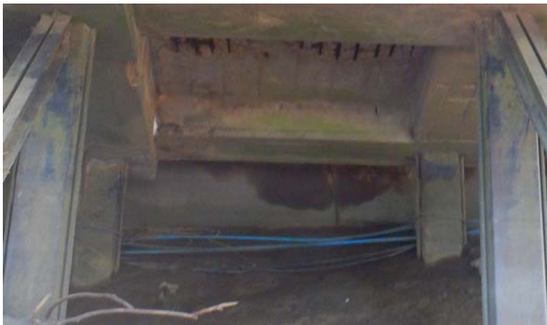
Photograph No. 10a
