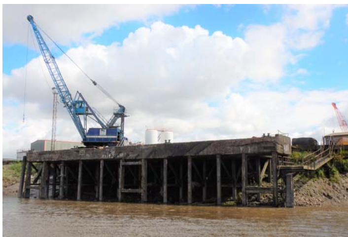
Gunness Wharf Main Jetty
