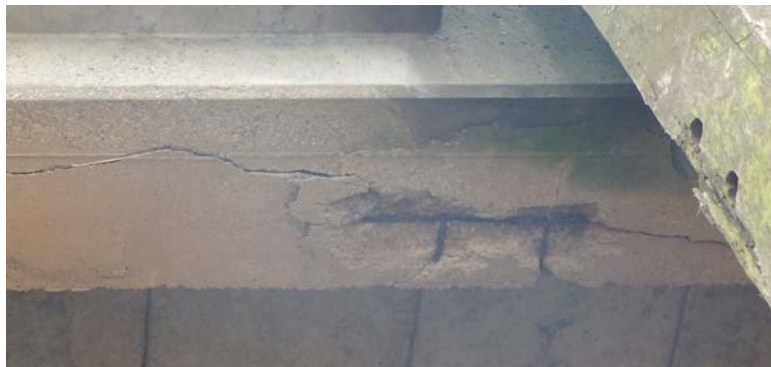
Photograph No. 12a
